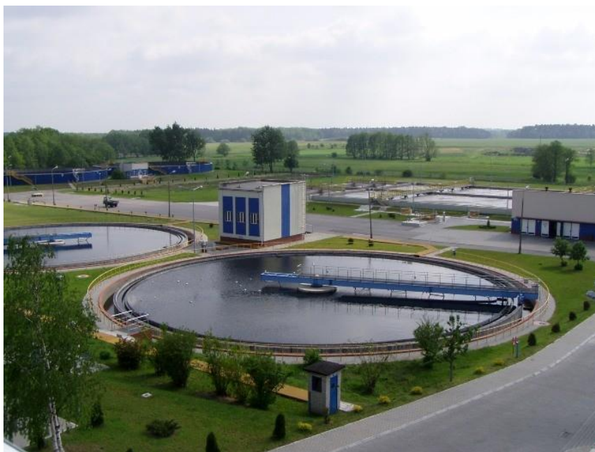
OPEN DIGESTION CHAMBERS
