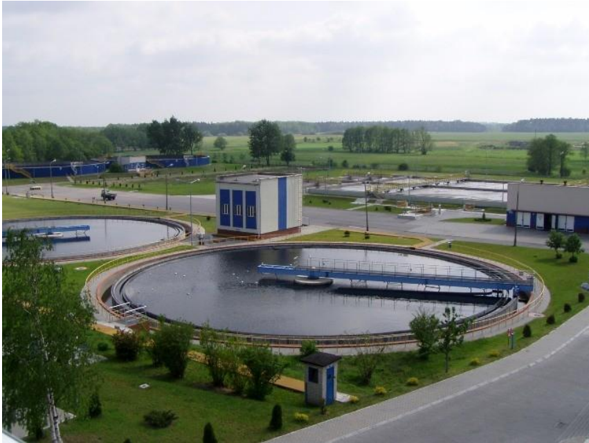
OPEN DIGESTION CHAMBERS
